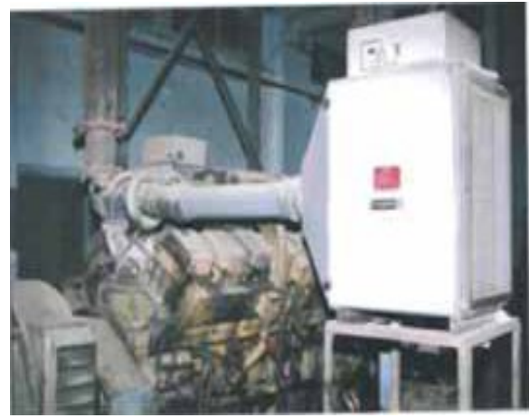
Air intake retrofitted with Electrostatic Air Filter
